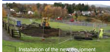
Installation of the new equipment
