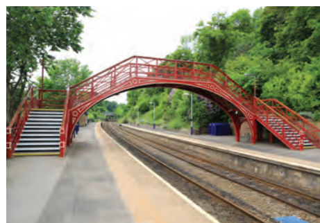
The newly repainted station footbridge at Stocksfield.
